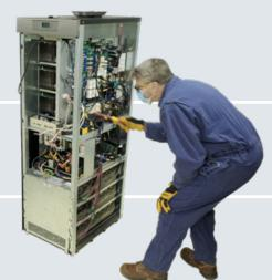
**9155 and 9355** UPSs have been manufactured from 2007–2021 and were designed for service longevity with modular field replaceable electrical components. With proper maintenance 9155 and 9355 UPSs can last for more than 10 years.
