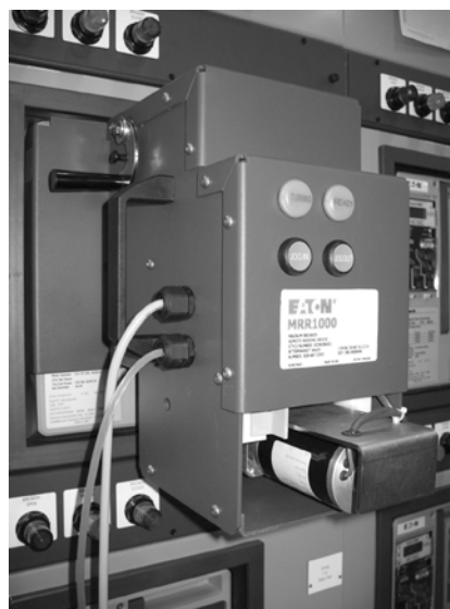
MRR1000 Connected to Magnum Breaker
