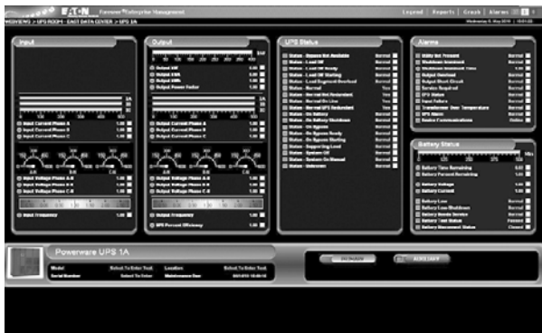
Eaton Powerware UPS-Primary View
