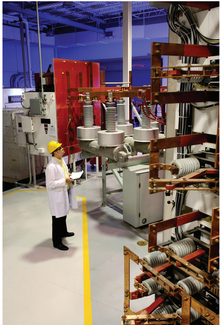
The Eaton Bussmann Division's Paul P. Gubany Center for High Power Technology is the electrical industry's most comprehensive facility for testing and certifying device and equipment SCCRs. Capable of performing electrical tests up to 600 volt three-phase, 300,000 amps of short-circuit current for meeting ANCE, ANSI, CE, CSA, ETL, IEC and UL testing requirements.
