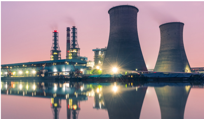
Utilities and power plants
